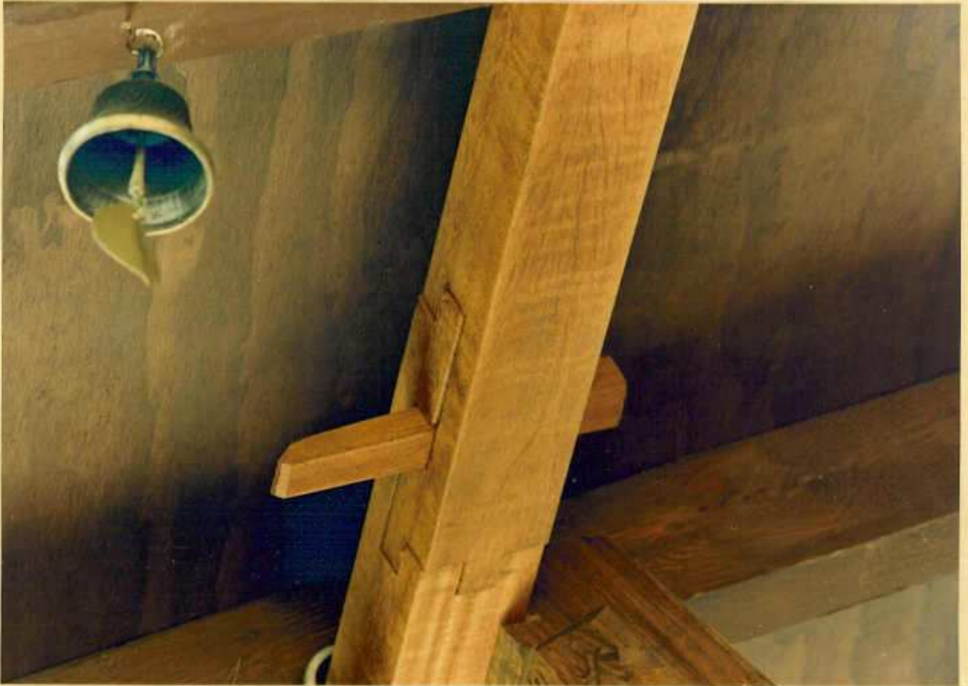
Traditional Join: a hand chiseled interlocking joint with wedge for longitudinal joining of strut purlin adapted for strength in compression and tension. A singing bell hangs above.
